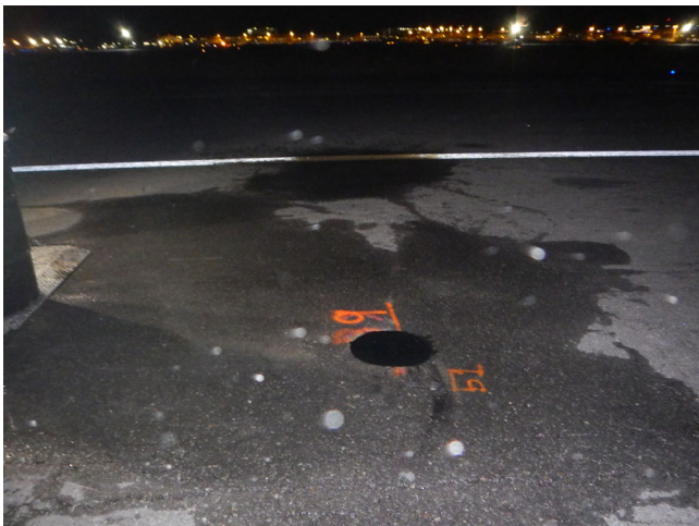
General Site Conditions around Boring B-9
