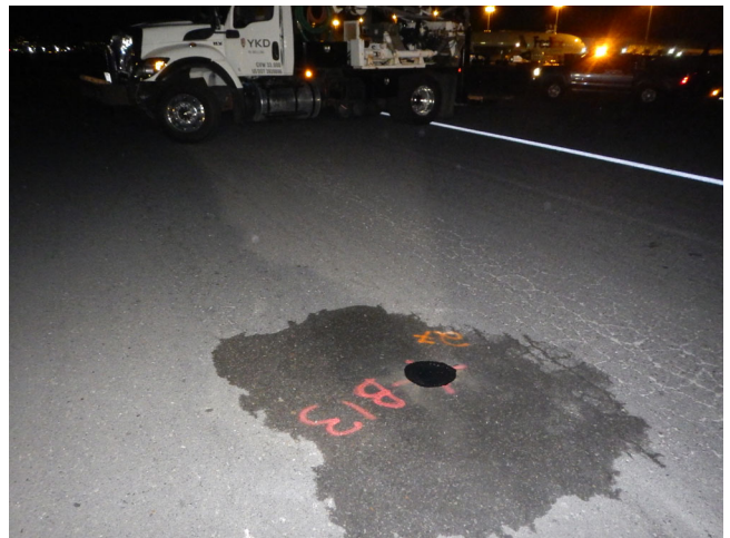
General Site Conditions around Boring B-13
