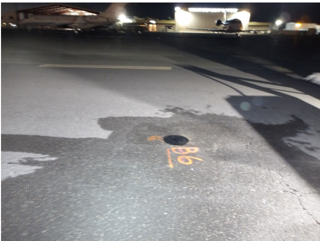
General Site Conditions around Boring B-6
