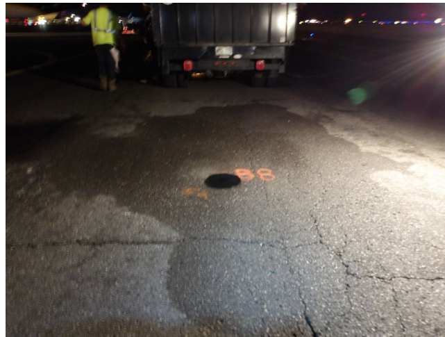
General Site Conditions around Boring B-8
