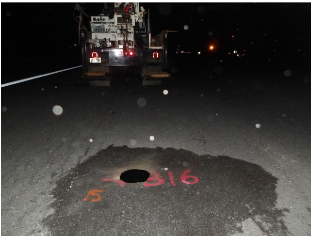
General Site Conditions around Boring B-16
