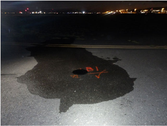
General Site Conditions around Boring B-1
