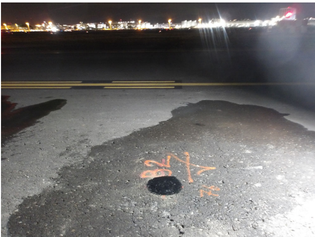
General Site Conditions around Boring B-2
