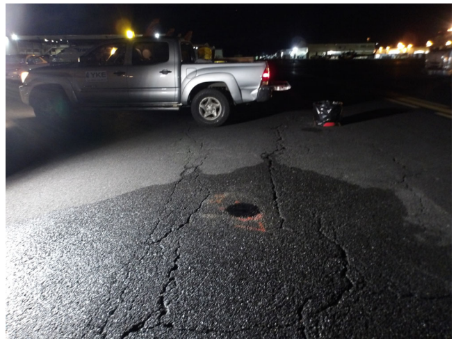
General Site Conditions around Boring B-7
