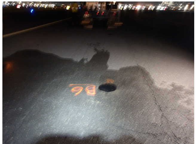
General Site Conditions around Boring B-6
