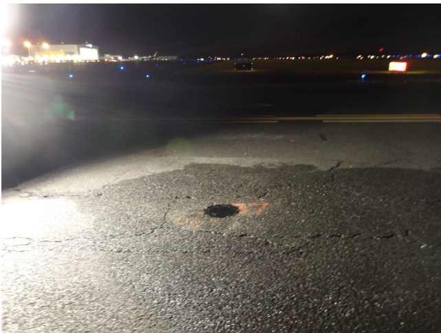
General Site Conditions around Boring B-7
