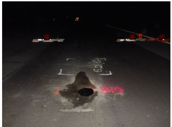
General Site Conditions around Boring B-19
