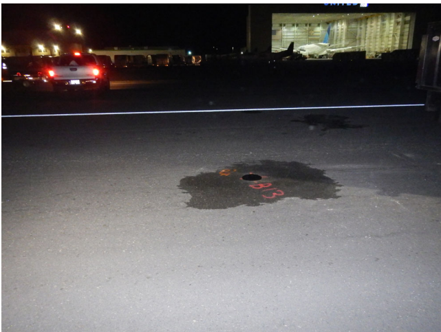
General Site Conditions around Boring B-13
