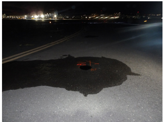
General Site Conditions around Boring B-1
