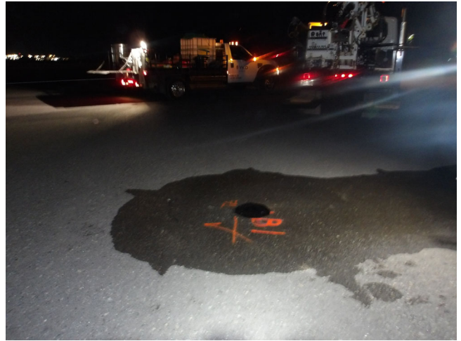
General Site Conditions around Boring B-1
