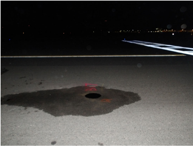
General Site Conditions around Boring B-17
