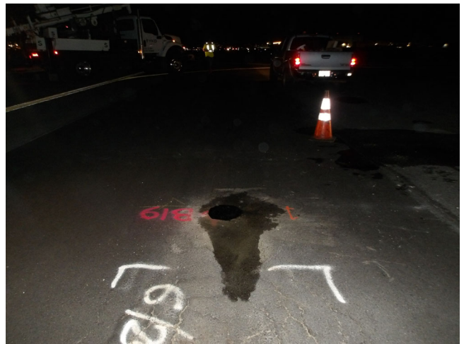
General Site Conditions around Boring B-19
