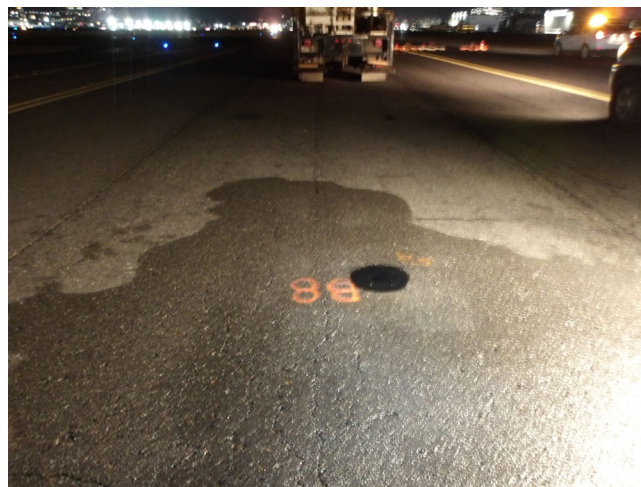
General Site Conditions around Boring B-8
