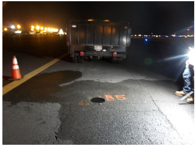
General Site Conditions around Boring B-5
