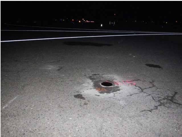
General Site Conditions around Boring B-15
