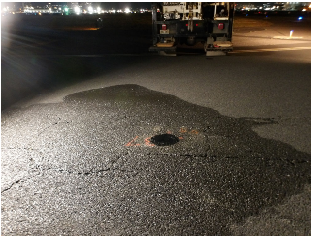
General Site Conditions around Boring B-7
