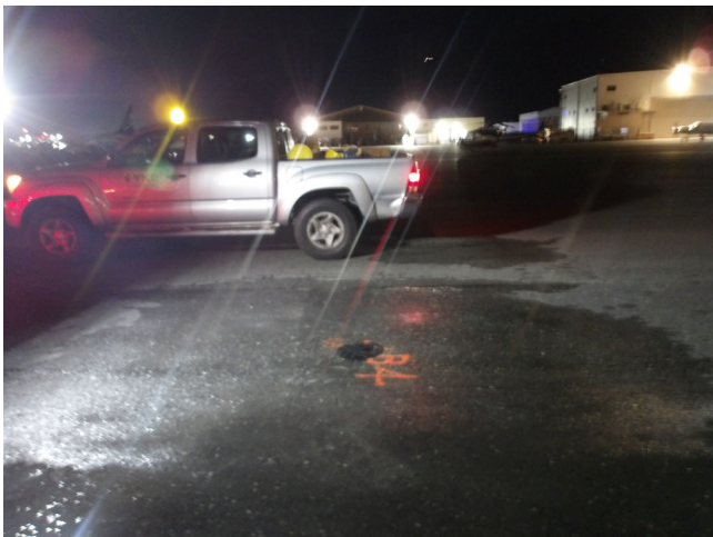
General Site Conditions around Boring B-4
