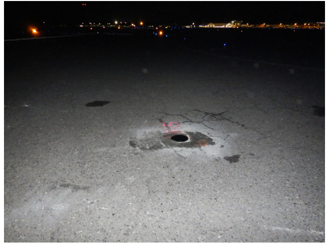
General Site Conditions around Boring B-15
