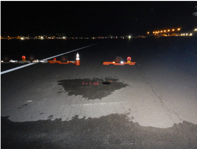
General Site Conditions around Boring B-14
