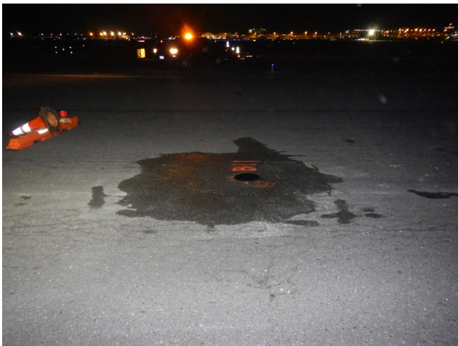
General Site Conditions around Boring B-11
