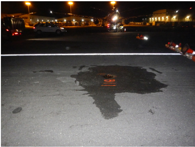
General Site Conditions around Boring B-11
