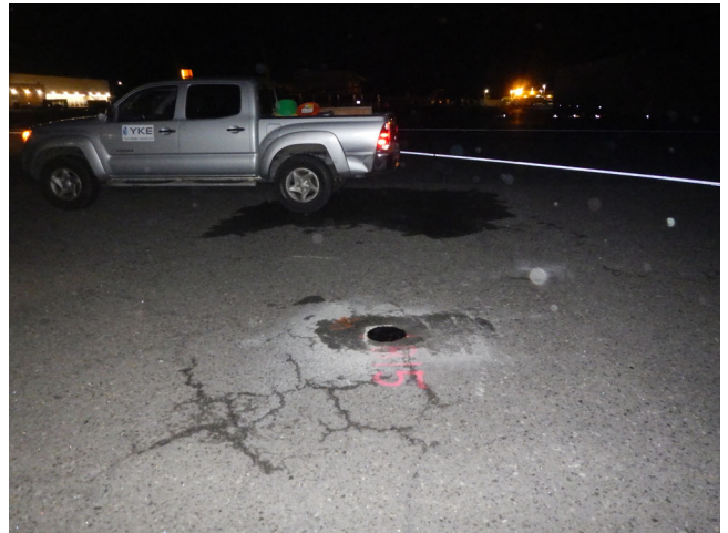
General Site Conditions around Boring B-15
